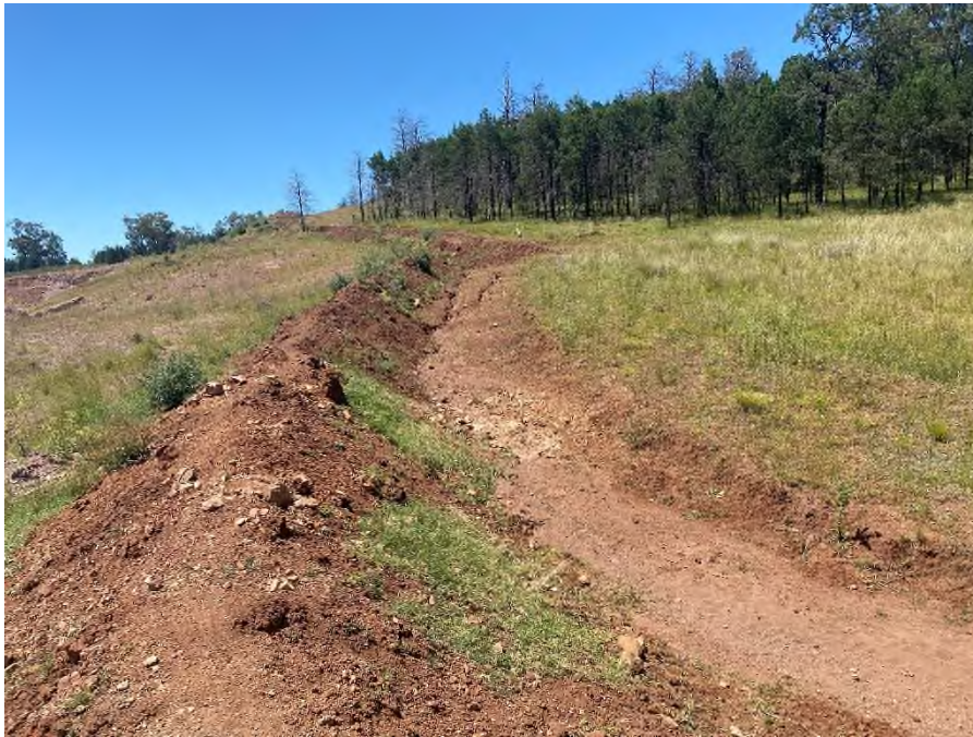
Photograph 4 , shows the cleared eastern side of the quarry viewed towards the north. An earthen bund wall has been constructed to divert runoff water away from the quarry pit to the south.
