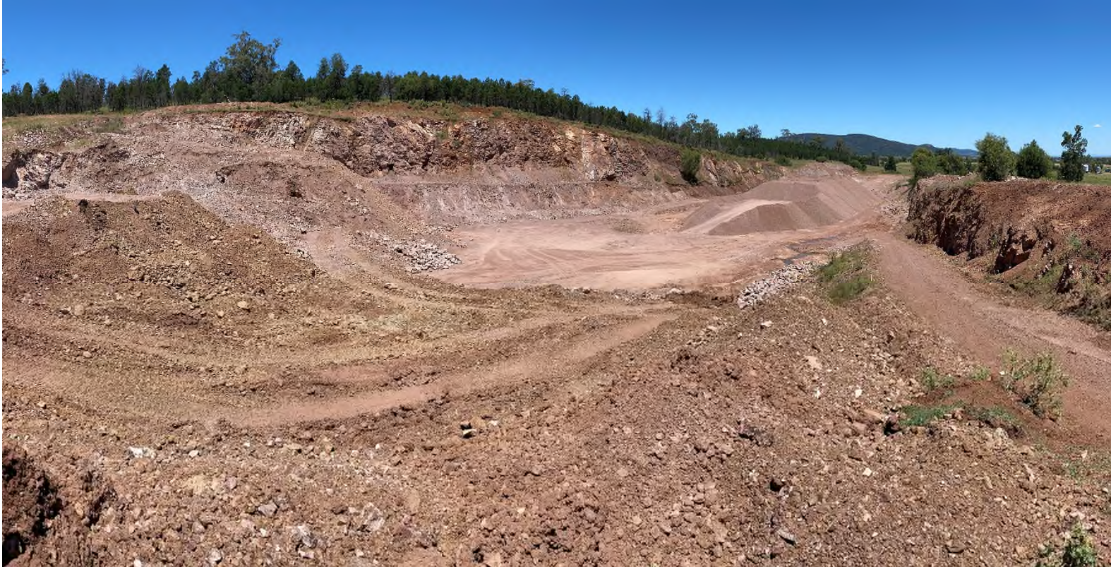
Photograph 1 , shows the existing Bolgers Pit and the extraction area in the north of the pit, left side of photograph, and current stockpile of crushed gravel material on southern base of the pit.
