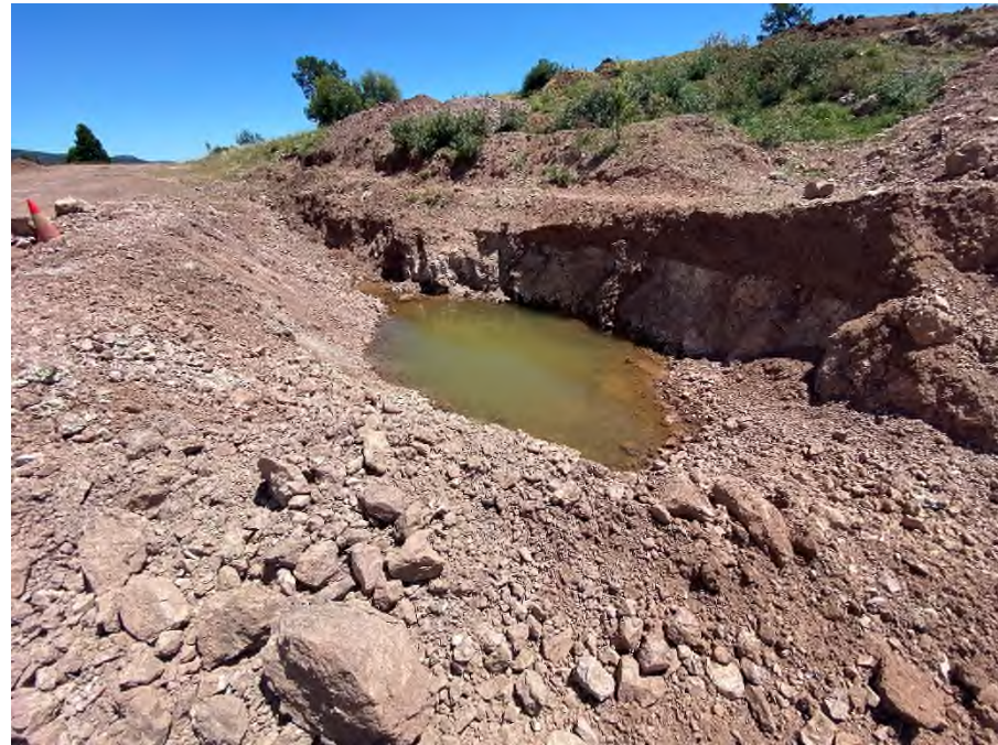
Photograph 5 , shows small diversion sump which has been excavated in the southwest corner of the quarry, viewed towards the south.
