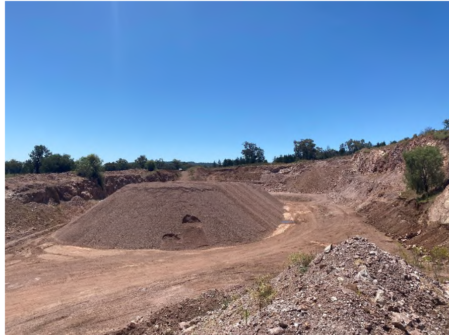
Photograph 3 , shows view inside the quarry pit, viewed towards the north.
